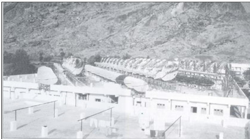
Arial views of Solar Cooker, which cooks food for 30,000 people on one hour, at Shantivan Complex, Abu Road.
